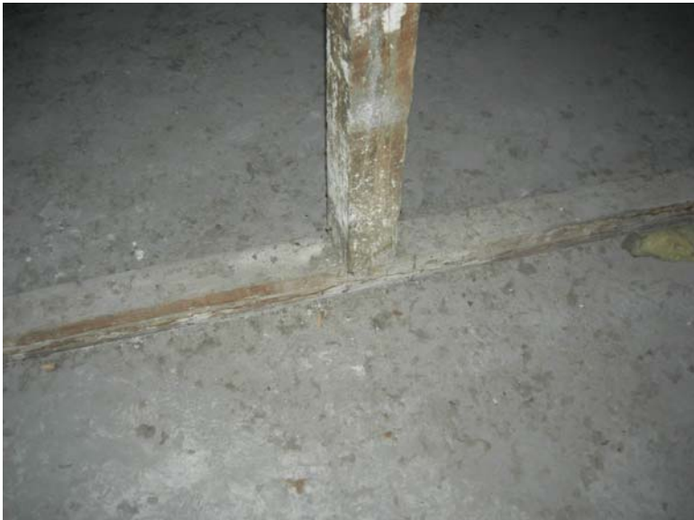
Photograph 02 Wood Post to Slab Connection
