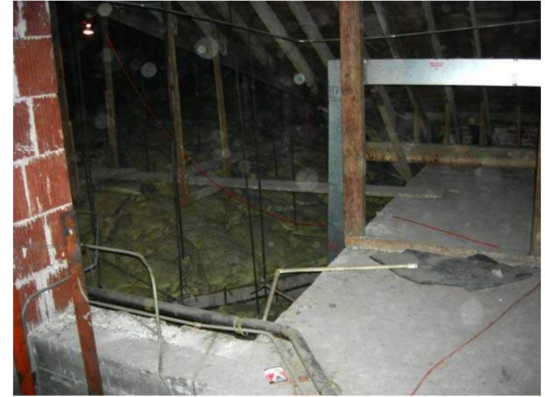
Photograph 06 Slab opening at Ceiling and catwalk
