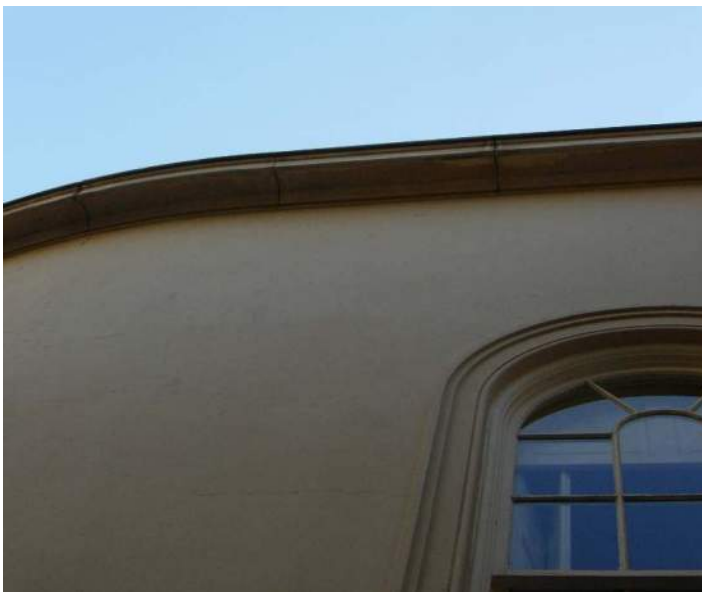
Image 2: Fascia/Soffit Water damage corresponding to downspout and scupper, roof area "C" North
