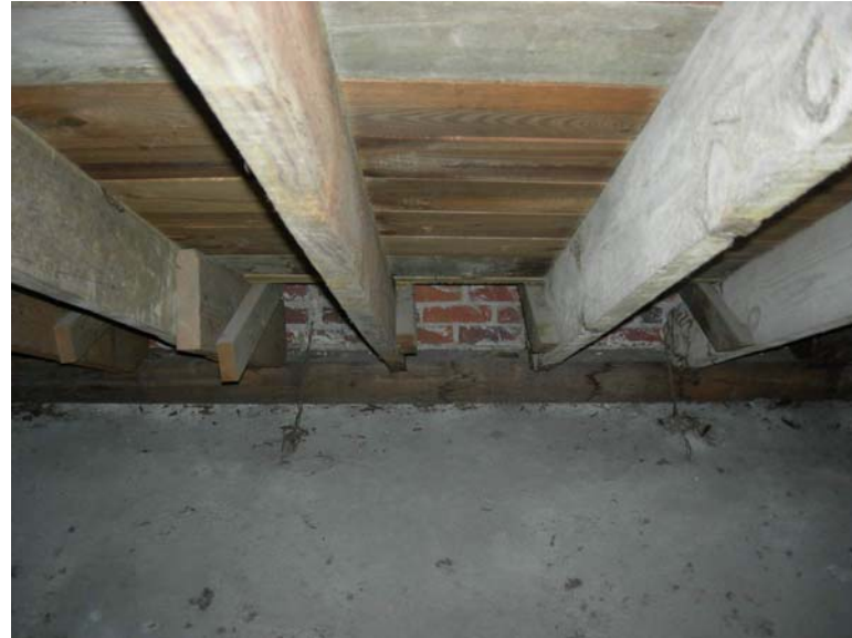
Photograph 03 Wood Sill to Slab Connection
