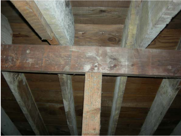
Photograph 01 Wood Beam to Post Connection
